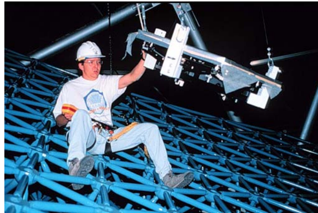
Lowering a segment into place on the truss.
