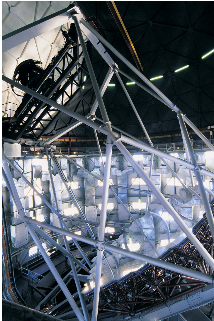
Figure 1: The completed SALT. The primary mirror array (91 segments) is seen to the bottom right, on top of the supporting truss, while the prime focus tracker and payload are seen at top left (in black), mounted on the “top hex” of the structure. The night time ventilation louvers can be seen in ring-wall, as can the daytime air conditioning conduits.
